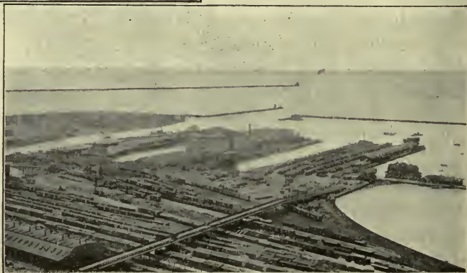
FIG. 66.—Breakwaters built at Chicago to form a harbor where ships may be safe from the waves.
